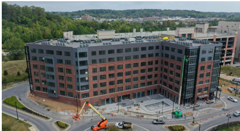
An aerial picture of The Met, our new 114 apartment high-rise in Owings Mills, MD.
